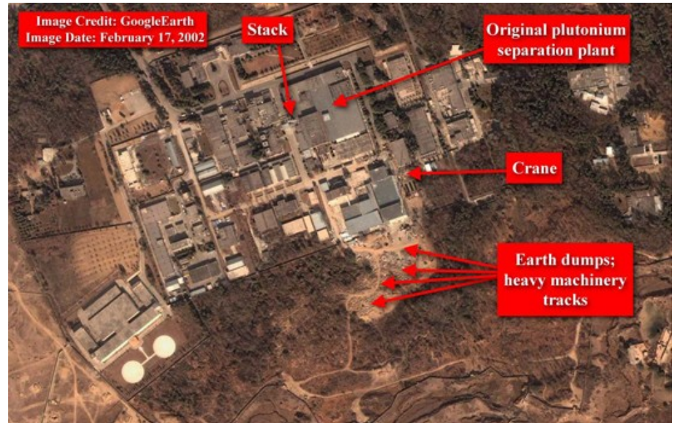
Plutonium Separation Plant Rawalpindi, Pakistan, Feb 2002
